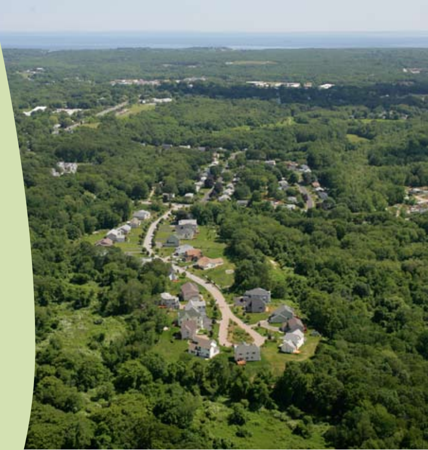
Example of low impact development: Jordan Cove in Waterford, CT © University of Connecticut
